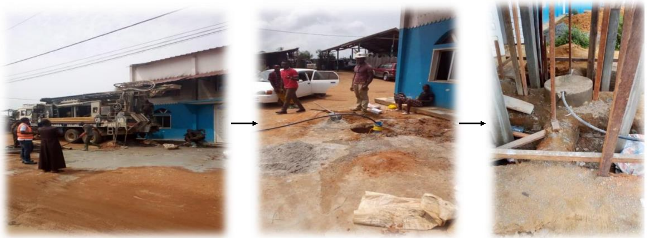
Construction of the borehole in the Newton Saint Thérèse parish
