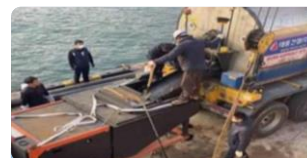
Injection of sandmastic mixture into the plant when underwater
