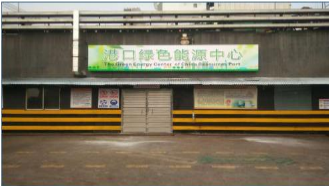
The green energy center of China Resources Port
