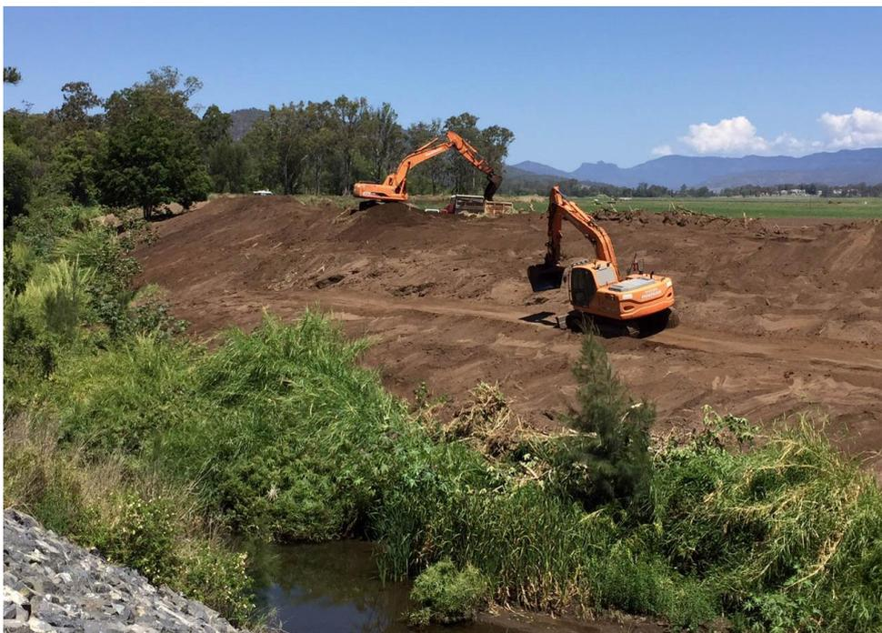
Stream restoration works comprised battering and stabilising the highly damaged banks of Laidley Creek. *Photo courtesy of SEQC Services.*
