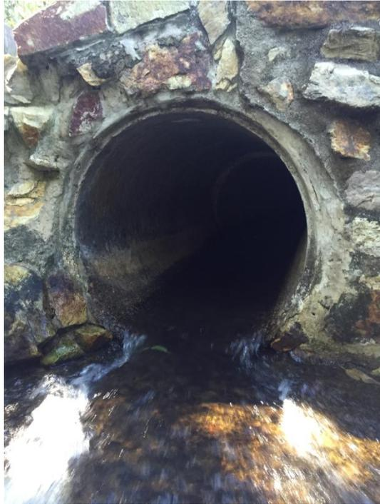
Clean stormwater runoff emerging from a collection pipe. The purpose of stormwater management is to ensure runoff is clean. *Photo courtesy of Planfuture.*
