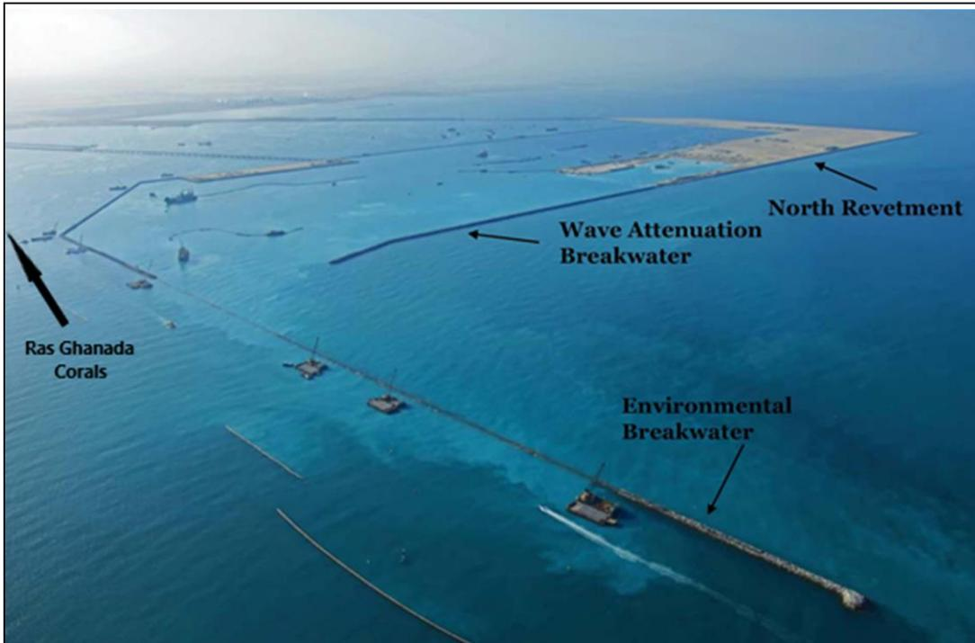
Figure 8 – Phase 1 under construction showing various breakwaters looking south
