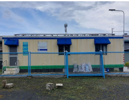
Establishment Carbon Neutral Facility
