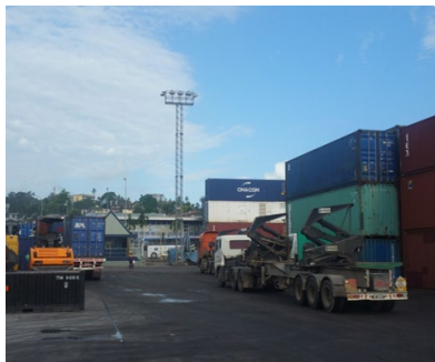
Port of Lautoka Yard 3 and Yard 4 Projects - Lighting Upgrades
