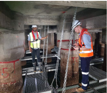
Wharf Rehabilitation Project - GTS installation Queens Wharf
