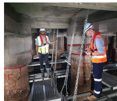
Wharf Rehabilitation Project - GTS installation Kings Wharf
