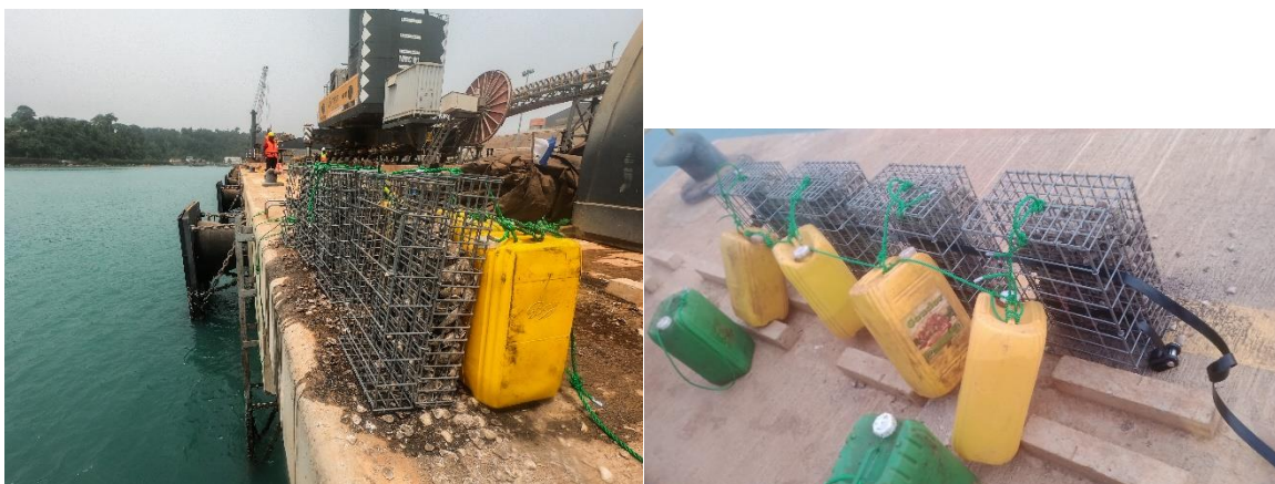
Figure 8 : Biohut pylon installation system
