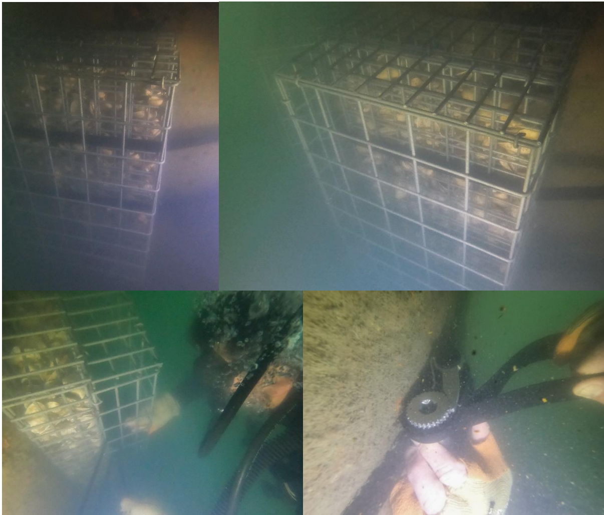
Figure 9 : installation of the Biohut on the pylons
