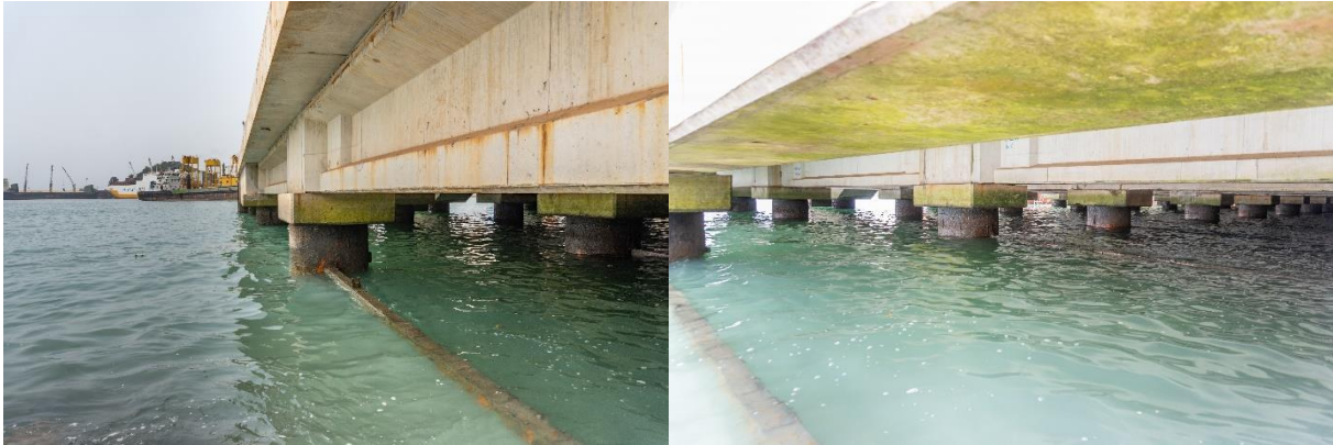
Figure 2 : view from the south of the pylons supporting the terminal
