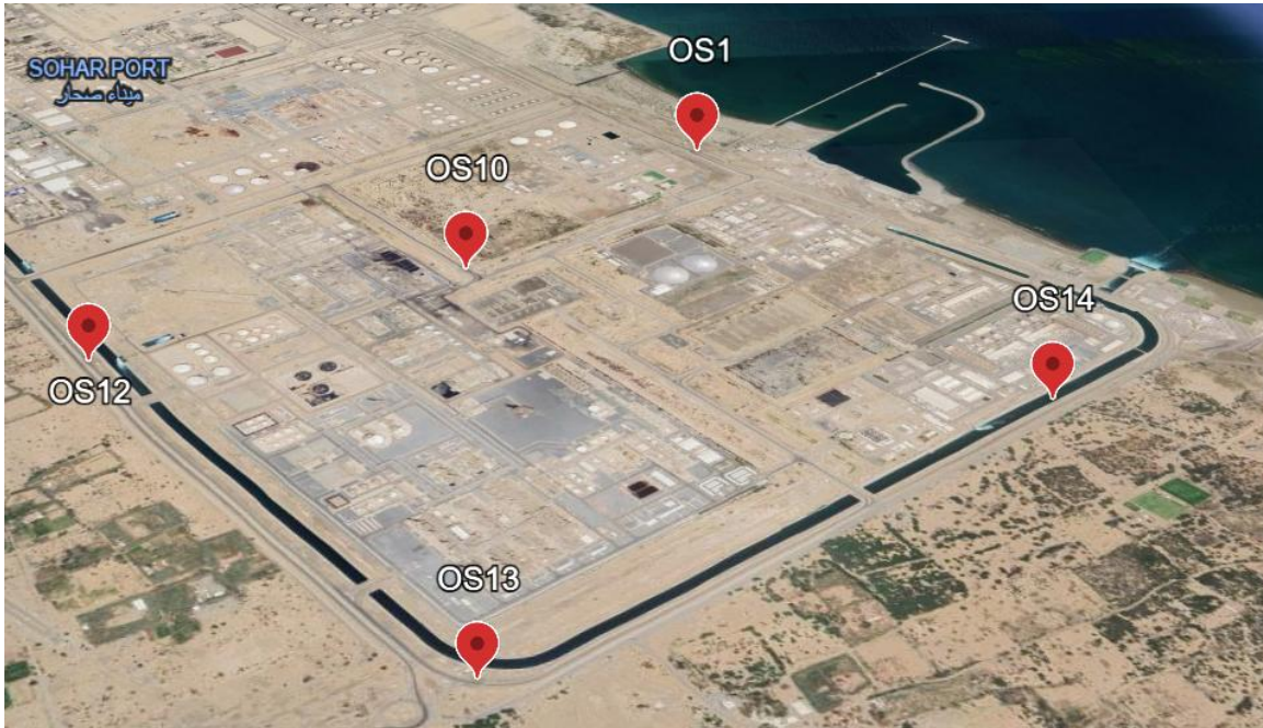
Figure 5 Bird view of the site with the Sohar Free zone in the southern part
