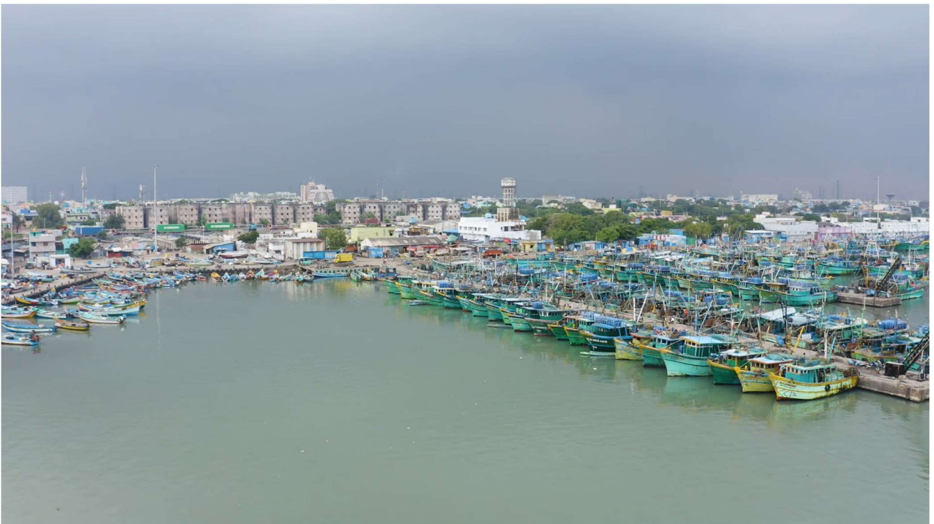
Chennai Fishing Harbour: Being Modernized by Chennai port
