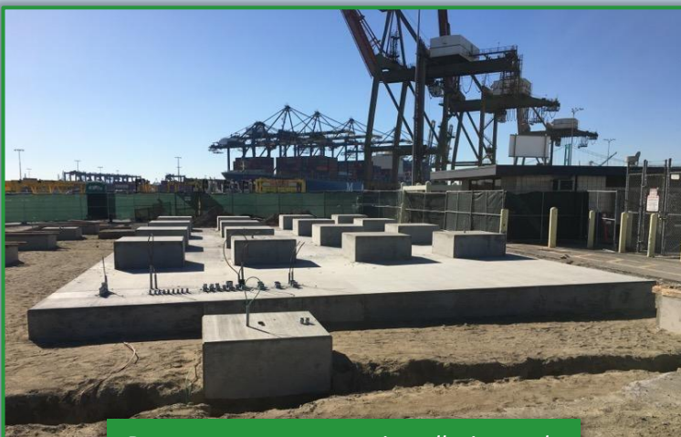
Battery storage system installation pads
