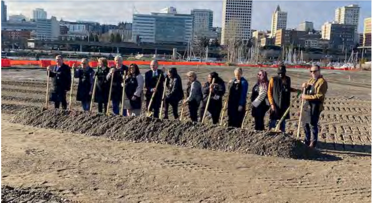
With shovels in hand, key partners in the project ceremoniously kicked off construction.
