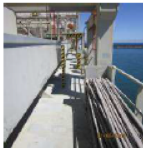
Lashing bars storage
