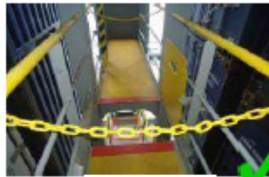
Bridge manhole with safety chain
