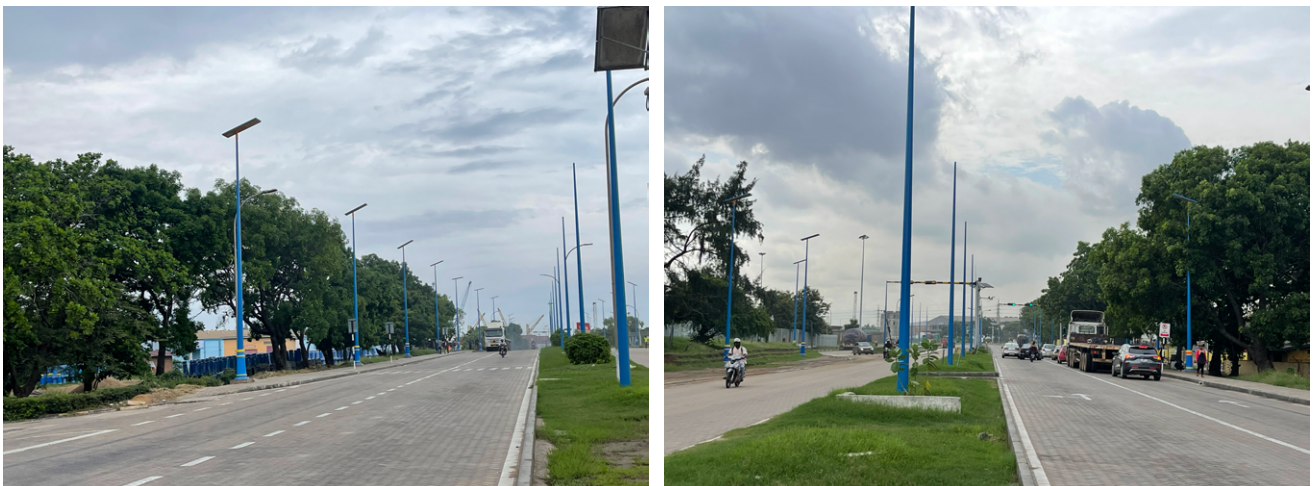
Installation of Street Lights within Port Environment
