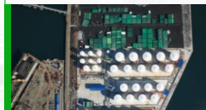
South New Port (Phase 1) fully opened
