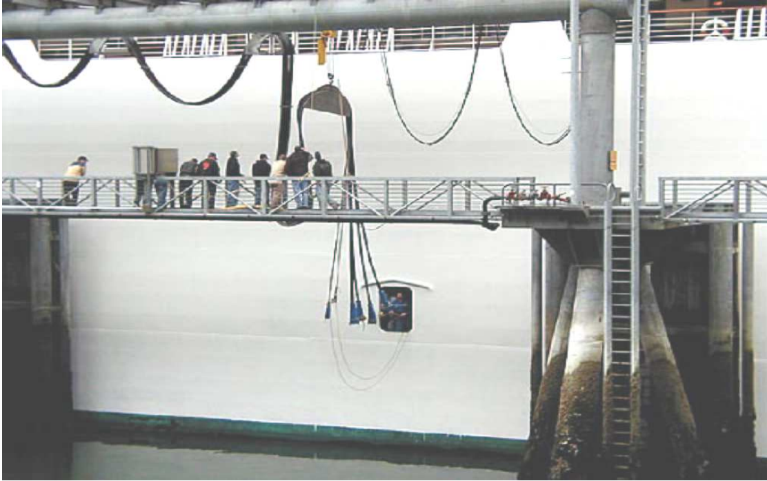
Figure III-3: Steel gantry festooning system at Juneau, Alaska
