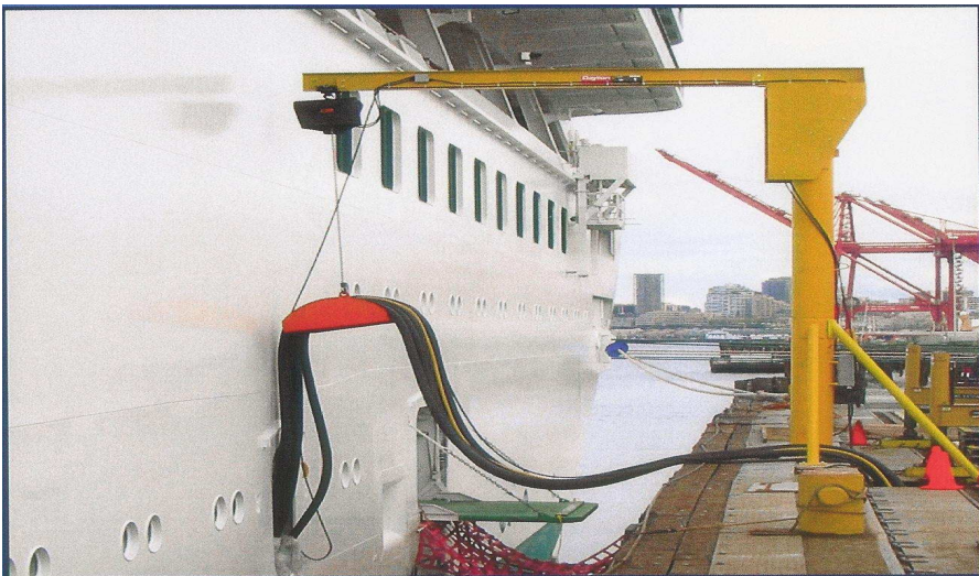
Figure III-6: Power cables at the Princess Cruises Terminal at the Port of Seattle
