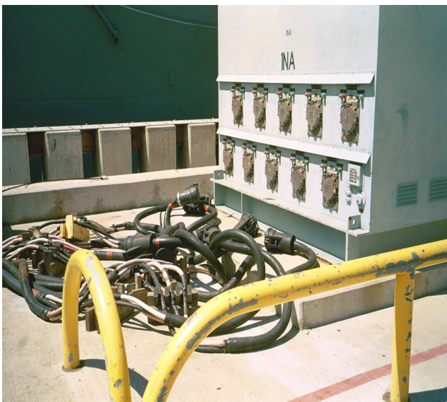
Figure III-10: Plugs stored at a substation at the San Diego Naval Station
