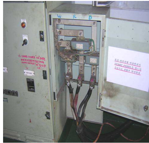
Figure III-8: Shore power connection on the Pacific Success at the USS POSCO facility.
