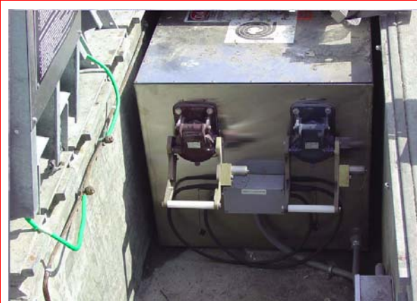
Figure B19 The electrical vault with two connectors located in the side of the quay.
