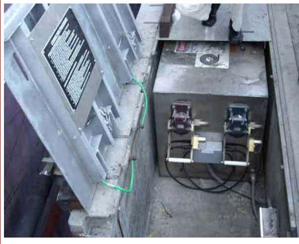
Figure D24 Connection box for double connection cables
