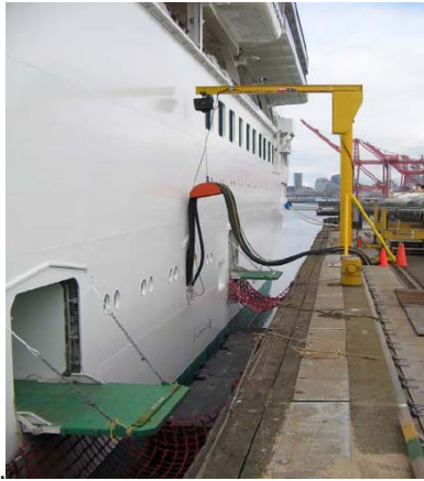
Figure B25 Cables are hoisted into position using a gantry.
