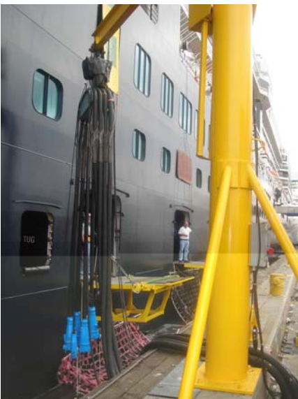
Figure B27 Cables are hoisted into position using a gantry. Each cable contains three cores (L1,L2,L3) and can carry 500 A per phase by 11 kV.
