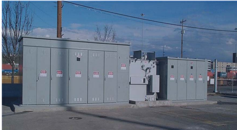
Figure B26 Transformer, main and secondary metering equipment. Transformer capacity is 16 MW. Primary voltage 27 kV. Dual service delivery (secondary) voltage 6.6 or 11 kV.
