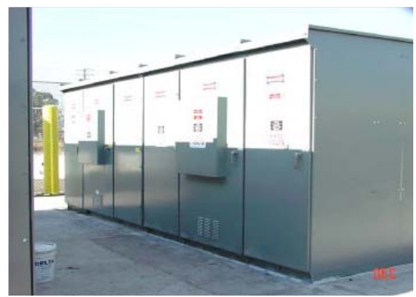
Figure B18 Main and Metering Equipment (6.6 kV)
