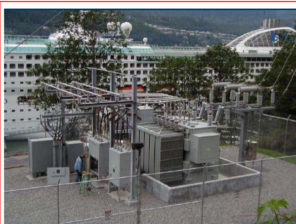
Figure B22 A dual-voltage transformer is used to step down the voltage from the local power grid to 6.6 kV or 11 kV.
