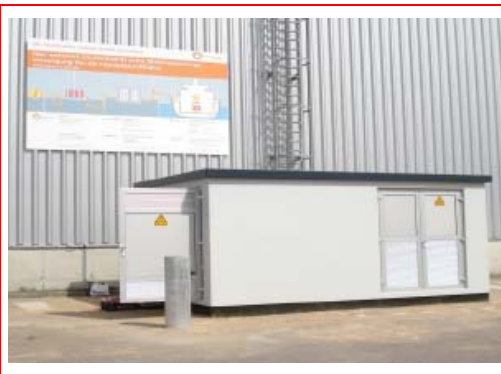
Figure B12 The transformer substation (10 / 6.6 kV 2.5 MVA) located on the harbour site next to the quay.
