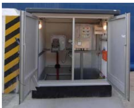
Figure B13 Cabinet with a 6.6 kV/50 Hz outlet enabling power to be obtained from the berth.
