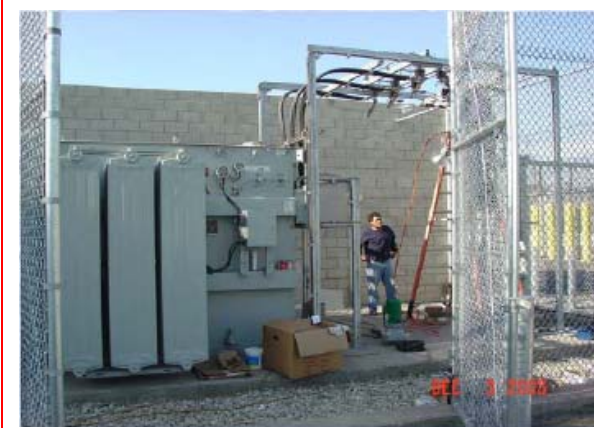
Figure B17 The utility transformer (34.5/6.6 kV 7.5 MVA) located on the harbour site.
