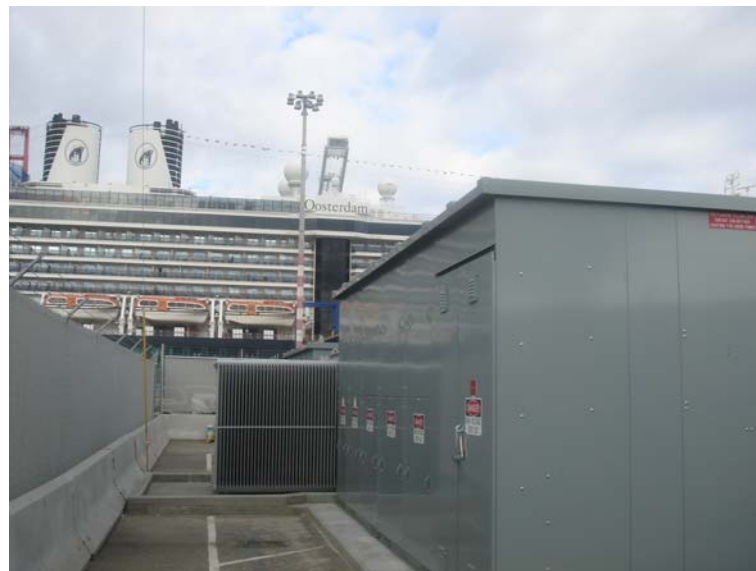
Figure B28 The pictures above show the incoming 27 kV power line and the substation, delivered and installed by Cochran Electrical Inc. (Main components such as the transformer and circuit breaker were provided by ABB.)
