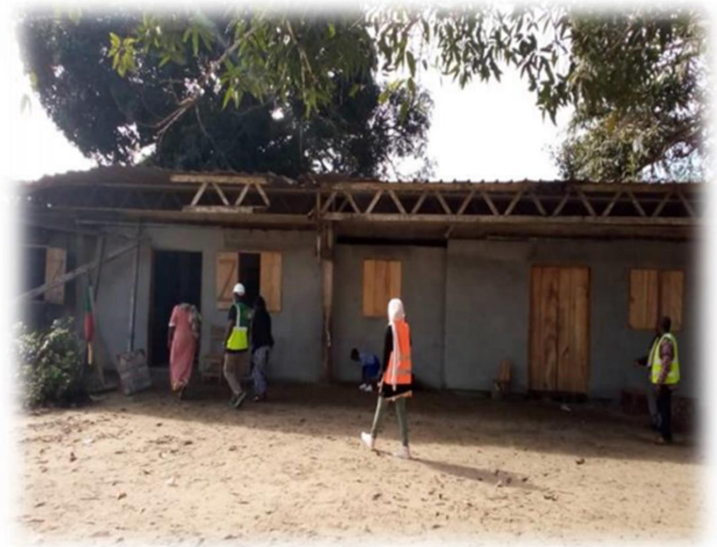
Two classrooms built already on the chosen site shown beside
