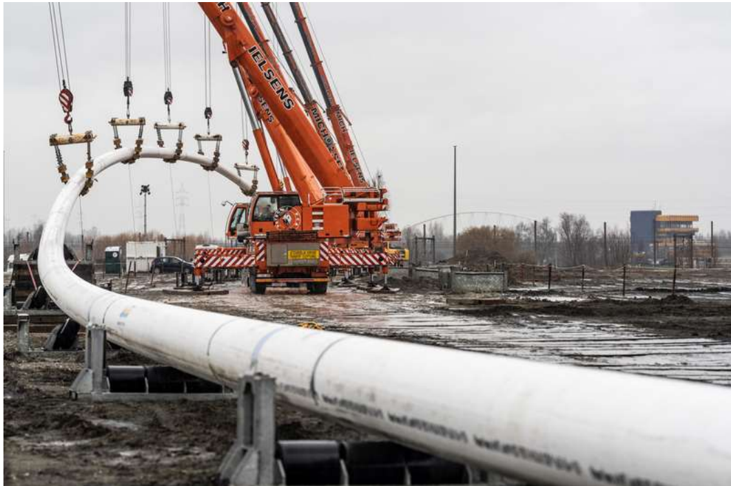
Building of the pipeline from Indaver to Boortmalt
