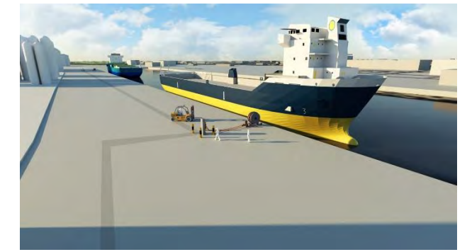
Figure 1—4 Shore power infrastructure on Mearns Quay. Ground scarring showing LV cabling route to shore power connection point
