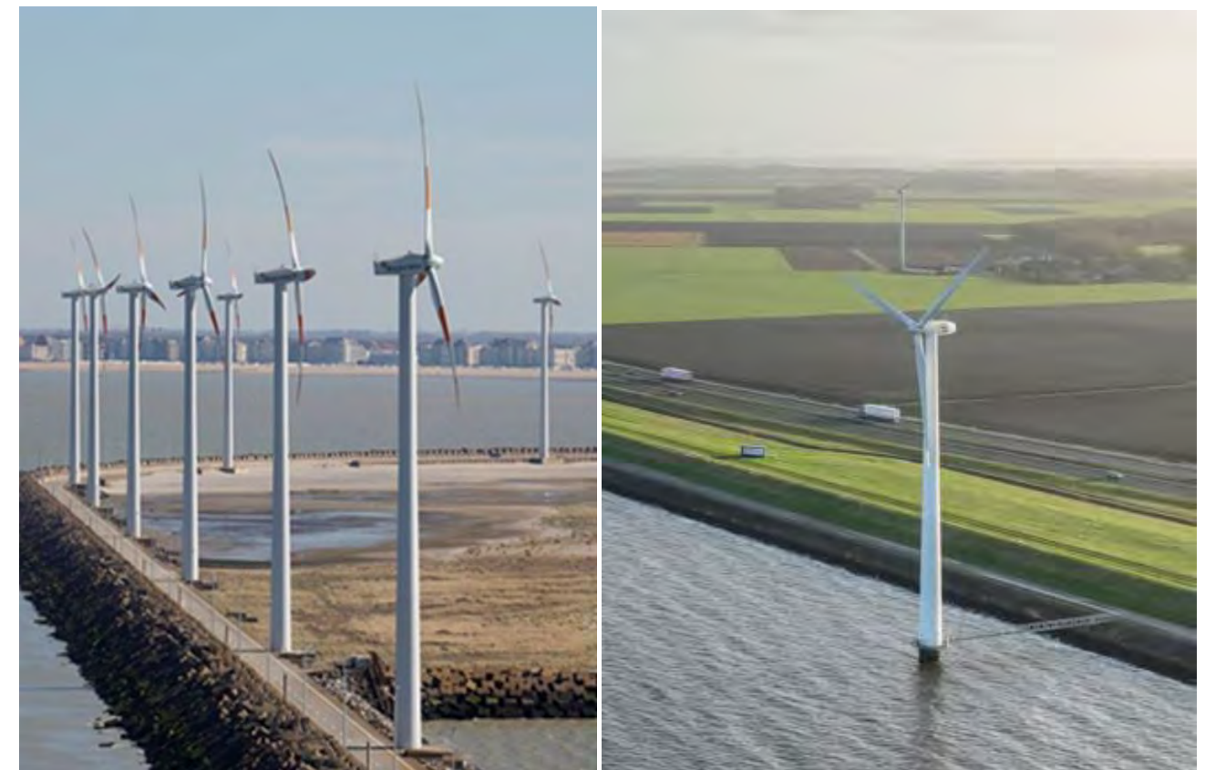
Figure 9—20 Example of wind turbines on a breakwater – Port of Antwerp-Bruges, Belgium (left) Example of (slightly) offshore wind turbine - IJsselmeerdijk, Netherlands (right)
