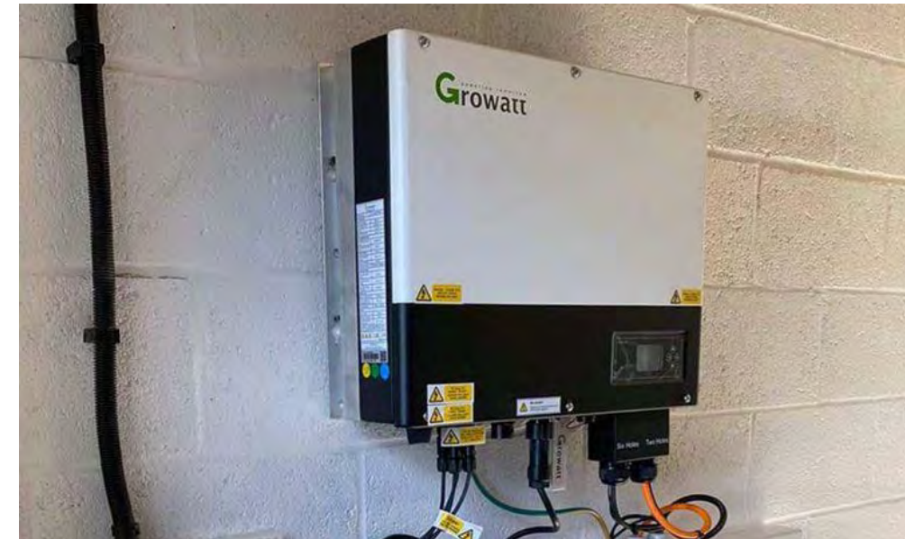
Figure 9—30 An example commercial/ industrial PV inverter
