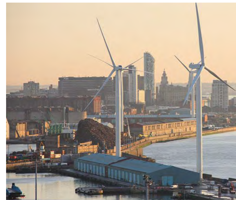
Figure 9—21 Example of wind turbines along a portside – Mersey Wind Farms, Port of Liverpool
