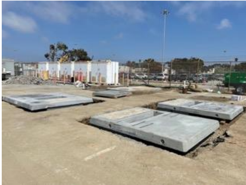
Photo Source: Port of Hueneme
