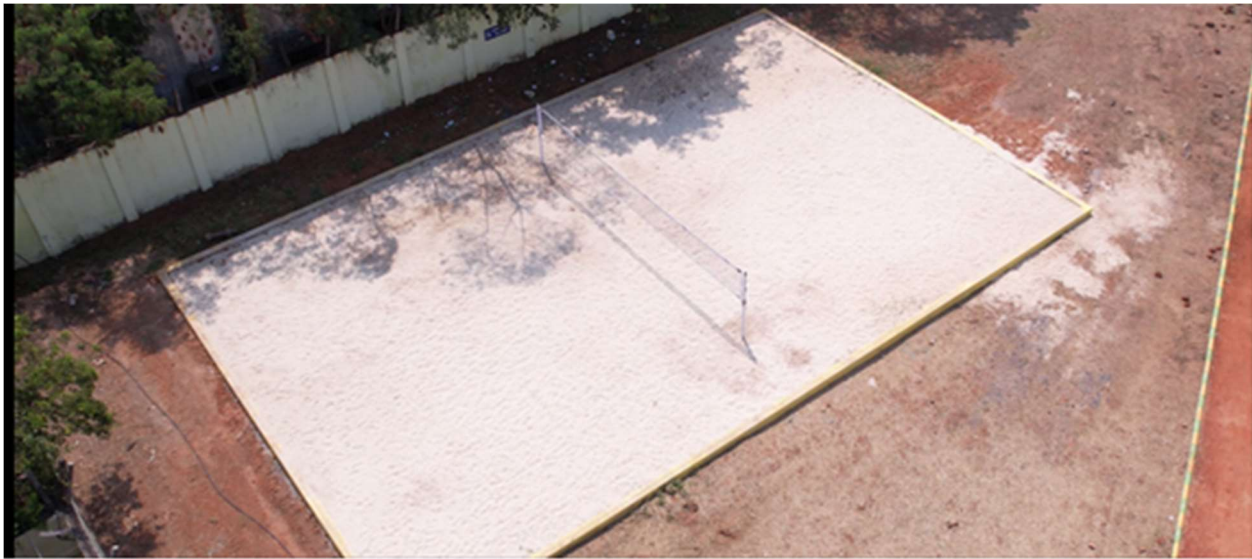
Chennai Port's Babu Jagjeevan Ram Sports Complex: Indoor Badminton court, Beach Volleyball court
