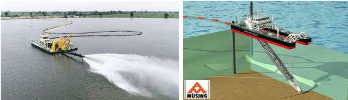
Picture 2: Typical dredging operation using the cut suction dredger Source https://jenkinsmarine.co.uk/services/dredging/ .
