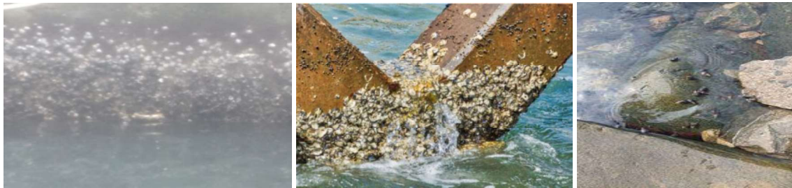
Picture 6: Barnacles on princess wharf and RHS, the common crustaceans
