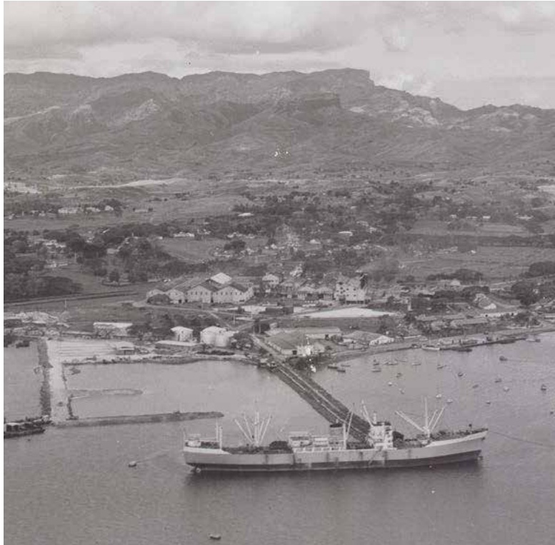
Aerial view of the Fiji Ports wharf in Lautoka with the Lautoka Sugar Mill in the background in the 1930s.
