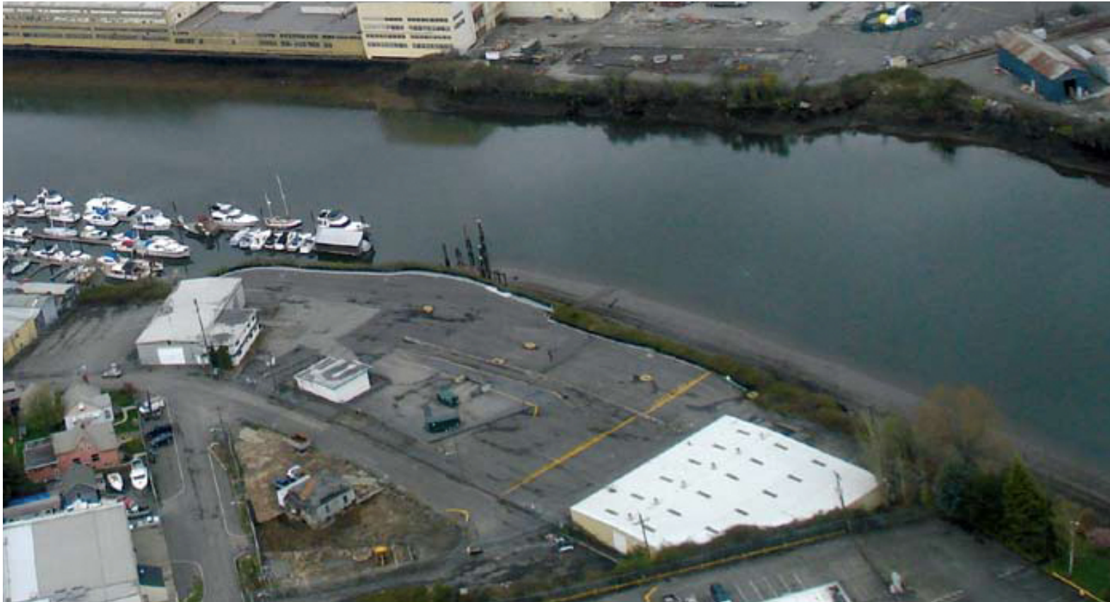
Terminal 117 project site, northeasterly perspective, with Dallas Avenue South and 17 th Avenue South in foreground. Former industrial buildings are present.
