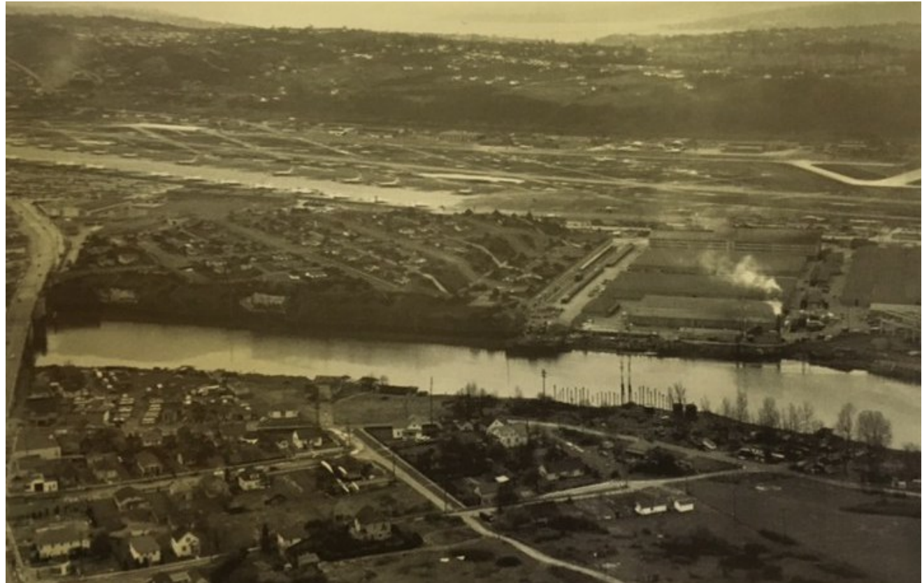
Terminal 117 project site, easterly perspective, with South Park Bridge at left and World War II era Boeing plant on east bank-line. Terminal 117 site is in foreground, water-ward of Dallas Avenue South/17th Avenue South/South Donovan Street right-of-way triangle. From Images of America: Seattle's South Park , photo courtesy of Theresa Lytle.
