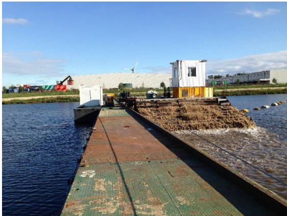
Fig. 2: Spray rinsing of sand (Ponton and aerial image)
