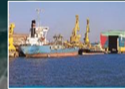
POSCO pier (raw materials, products)
