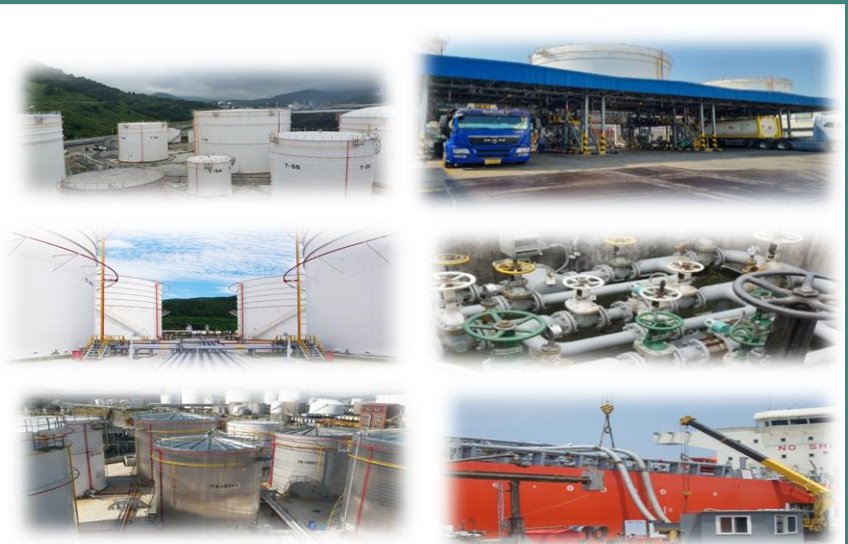
Storage of liquid cargo
