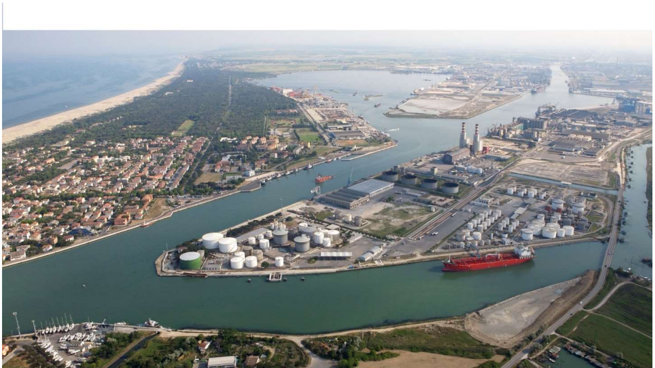
Figure 4-1. Port of Ravenna
