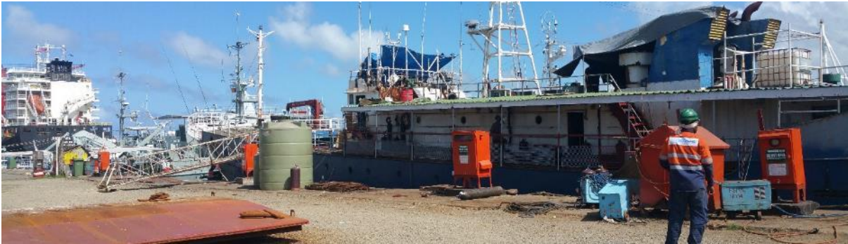
Figure 1 FSHL has already installed shore power (the orange boxes along the wharf)
