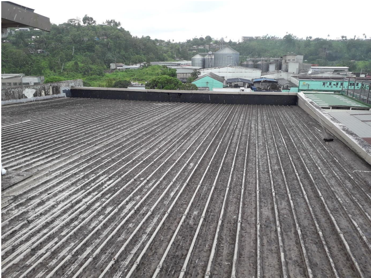
Figure 8 The rooftop of Muaiwalu House, and the rooftop of Muaiwalu waiting area are suited to the installation of solar PV.
