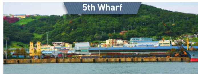
Length 802m Operator Publicly owned Cargo Steel, scrap metal, and miscellaneous goods
