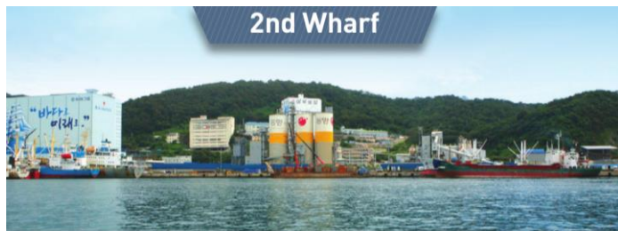
Length 1,062m Operator Publicly owned Cargo Frozen and general cargo steel, cement and sand
