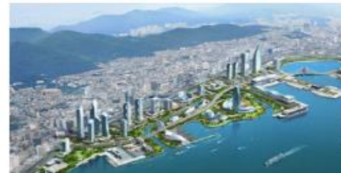
Construction of port redevelopment project and marina facilities
