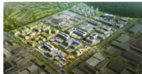
Construction, management and operation of Busan Port Distripark
