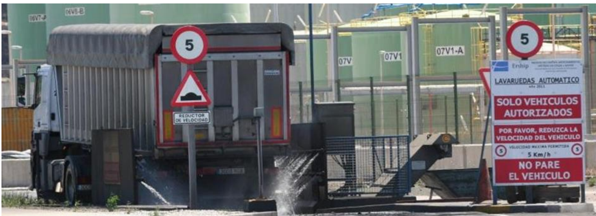
Automatic wheels cleaner installed at the Bulk Goods Terminal to reduce dust emissions generated by goods transportation
