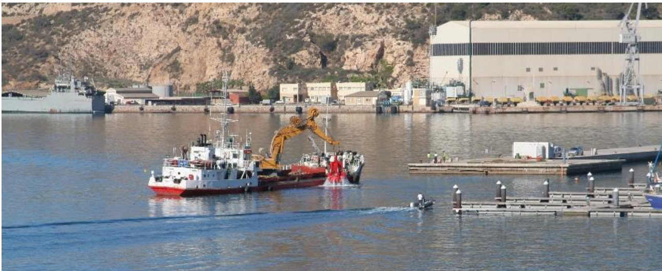
Dredging works to extend the Cruise Ships Terminal at Cartagena Port
