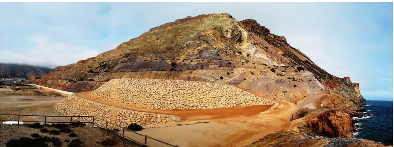
Slopes consolidation and plantation
