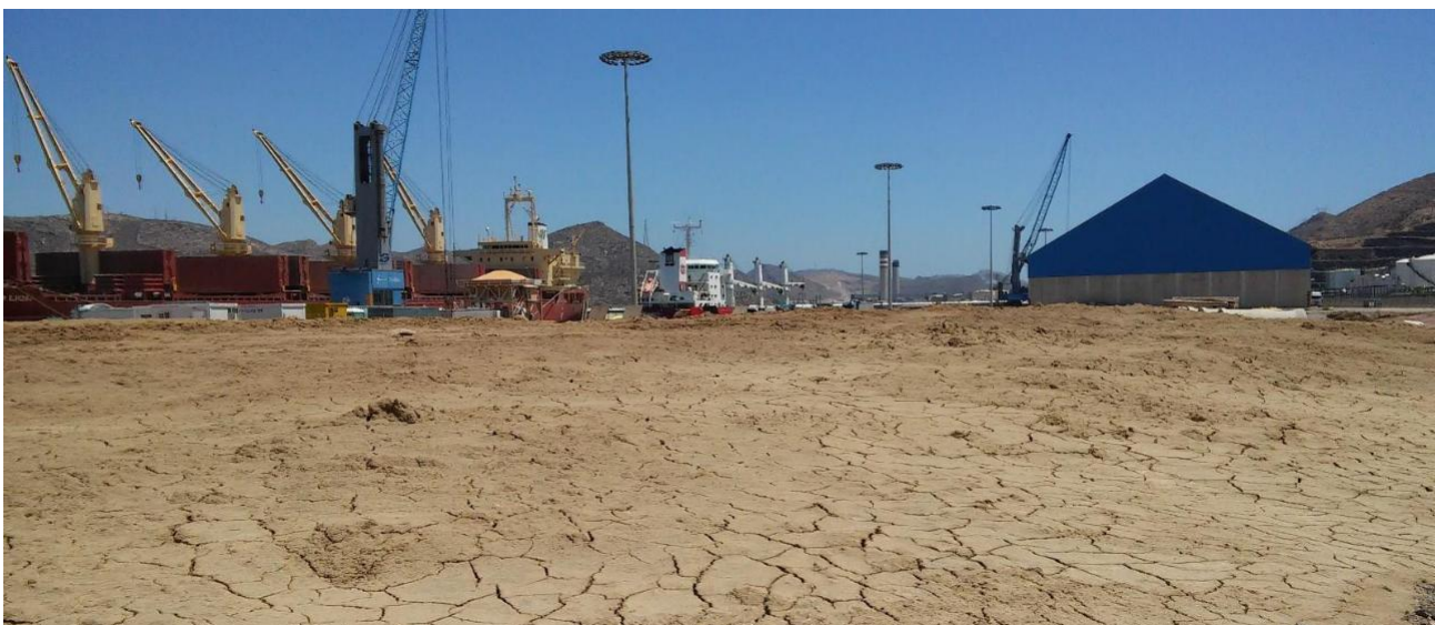
Dredging material deposited at Escombreras's dock extension before being managed as Non-hazardous waste
