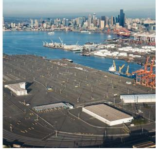
Plans to redevelop Terminal 5 in Seattle include dock and power upgrades and berth deepening to simultaneously handle two 18,000-TEU vessels.
