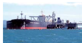
Raw material Pier& CTS wharf 7 berths [250,000 × 2/ 200,000 × 3/70,000 × 1/30,000 × 1]
