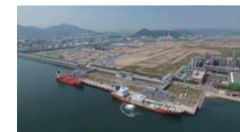
Petrochemical terminal 2 berths [10,000 × 2]
