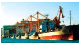
Steel Products wharf 11 berths [50,000 × 1/30,000 × 4/ 20,000 × 1/5,000 × 5]
