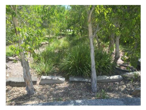
An installed WSUD at the Port. Sediments and pollutants in stormwater running off hardened areas (e.g. concrete) are intercepted by the vegetation, which also boost the landscape amenity of the Port.
