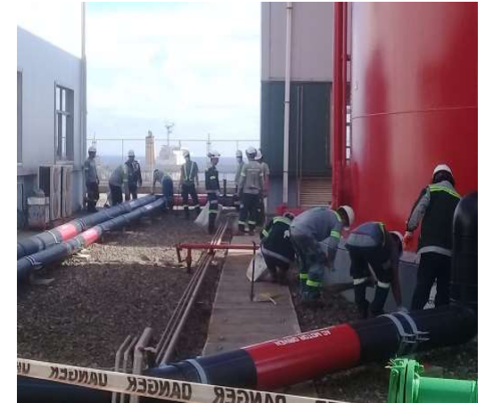
Fire Water Tank
