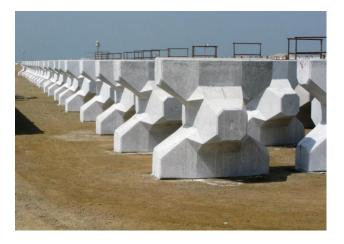
Figure 7 - Accropode<sup>™</sup>units stored ready for transport to the breakwaters.
