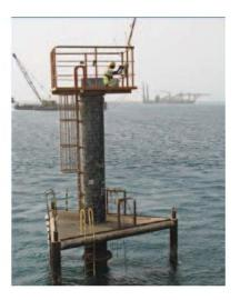
Figure 5 - location of monitoring equipment and one of the permanent stations installed.
